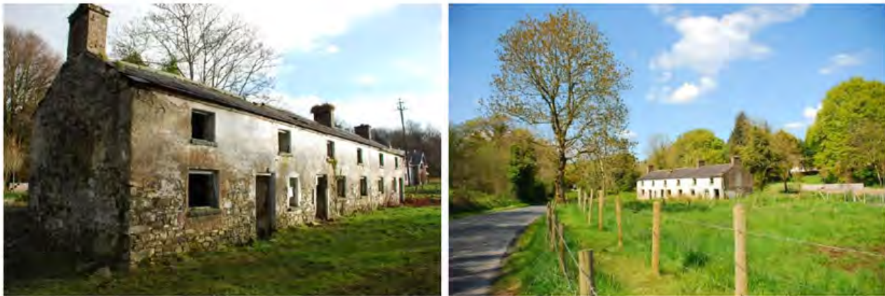
Above: Dundrum Road, Tassagh, B1 Listed Terrace, protected initially by BPN © DfC
